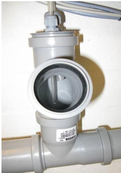
When the AI waste tube (ø10) is fixed in the drain it is important to keep the end of the tube visible through the overflow but still above the highest possible water level. Furthermore it is important that the ø10 tube has a positive slope all the way from the AI to the drain. The mainline tube (ø4) should be fixed with the end below the overflow (to prevent splatter).
