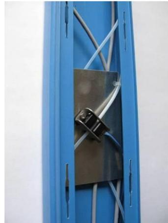
If possible BD1 should be in a vertically mounted cable trunk. Horizontally mounted cable trunks can be used but then the cable trunk opening must point outwards and not upwards! This is to ensure that the tube and the sensor can be mounted in a way so that the fluid in the tube will flow away from the sensor
